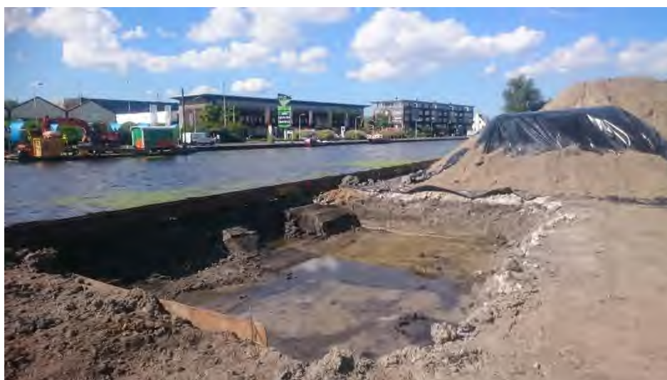
Vlek 4, foto 1 (ontgraving)
