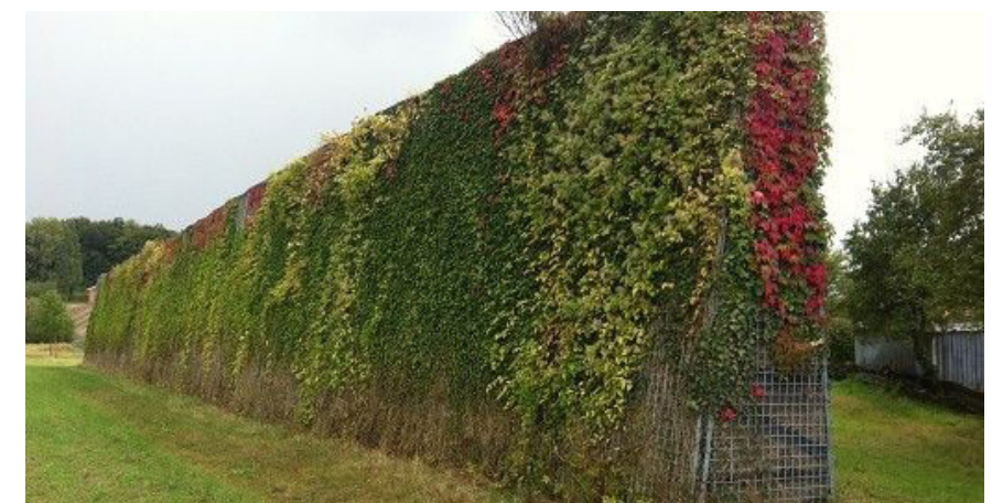
Kokosscherm (Greenwall construct) - langs weg/spoor
