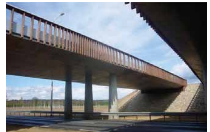
Viaduct Greenportlane, Venlo (NL)
