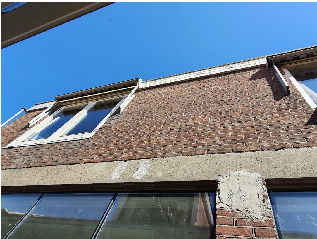
Plangebied Scharloo 19, Brielle, detail dakrand
