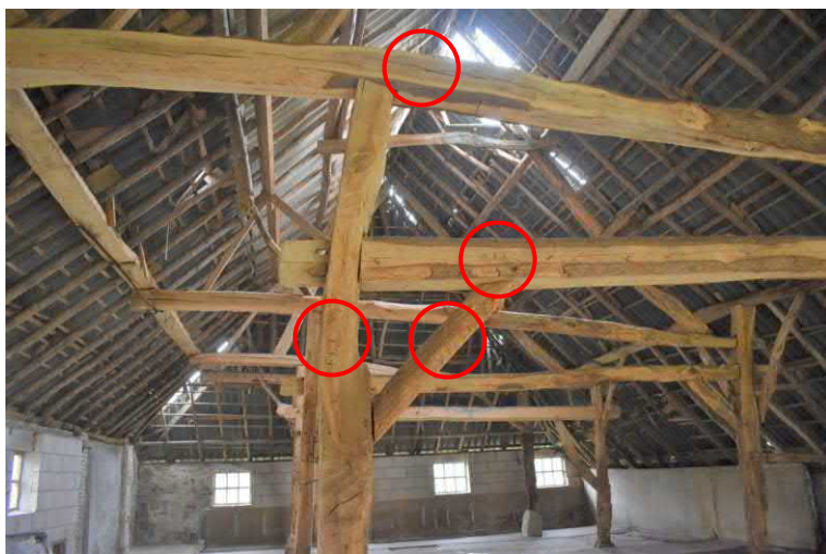
Telmerk IIIV in rechterzijbeuk.
