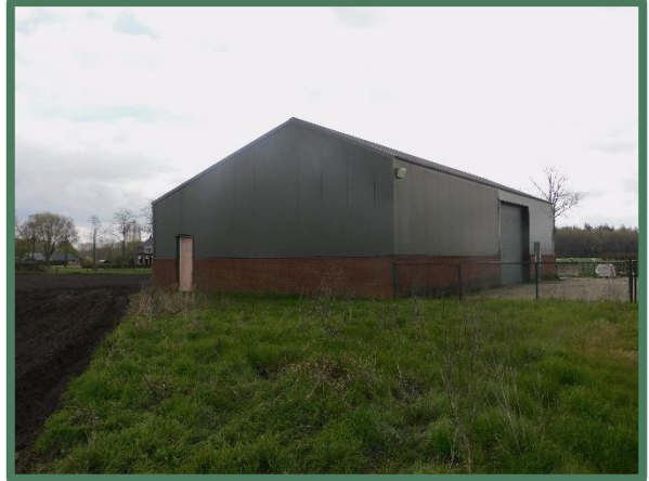
Te slopen loods
