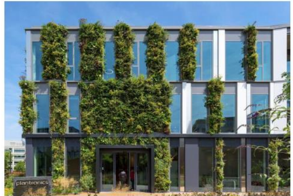
N4. Plantronics Hoofddorp William McDonough & Partners i.s.m. N3O architecten
