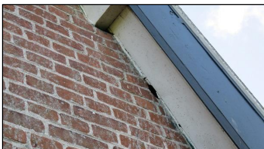
Foto 11. Opening in de dakrand
