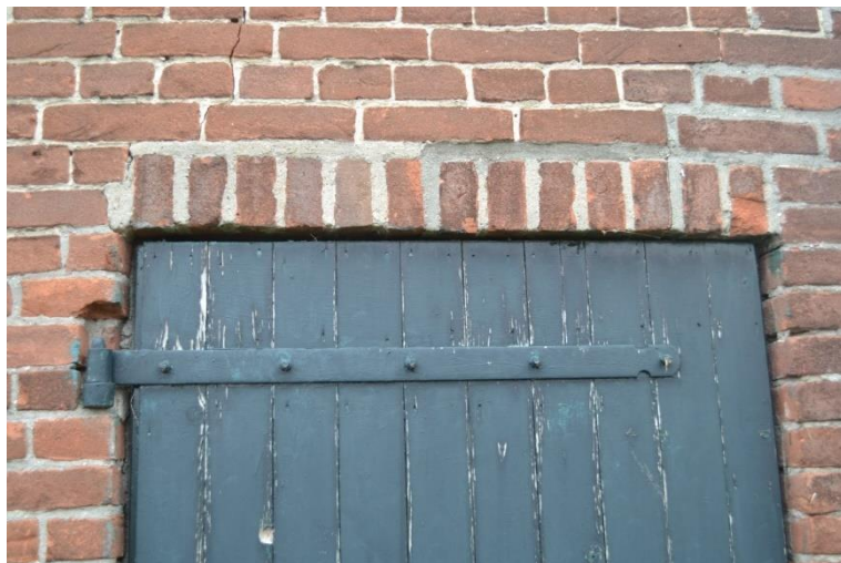
Later aangebrachte houten staldeuren.
