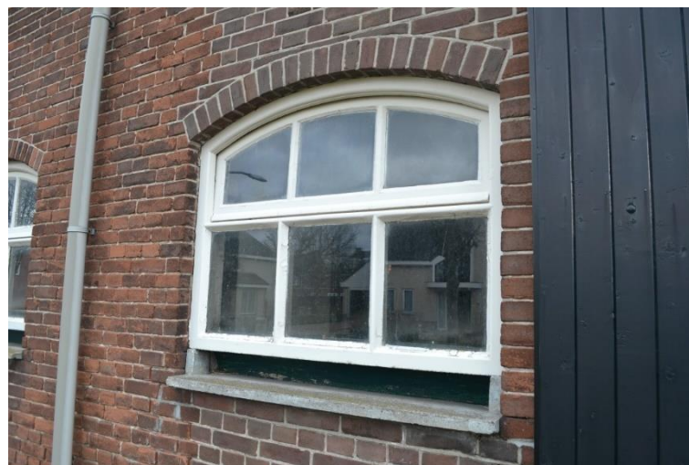
Later aangebracht betonnen stalvensters.
