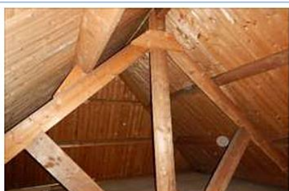
Houten gordingen en houten dakbeschot
