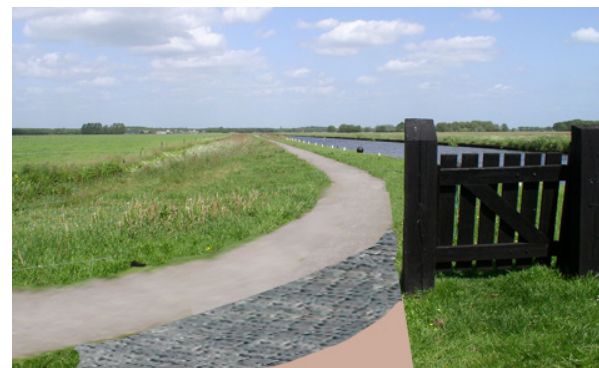
referentie markering bypass
