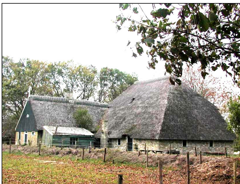
Wieringer boerderijen (bovenste foto: website In Pago Wirense)
