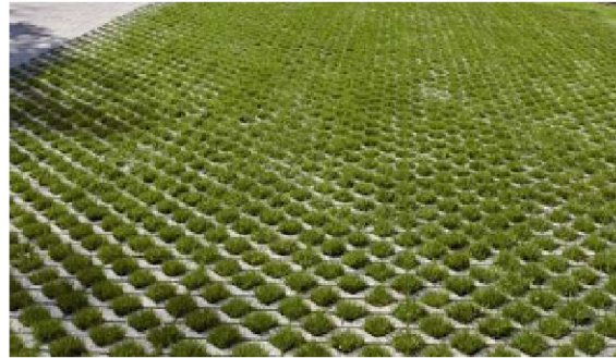
Referentie, half open bestrating parkeren, grasbetonstenen
