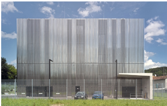
FFBK Architects Data Storage Centre Basel Basel, Switzerland
