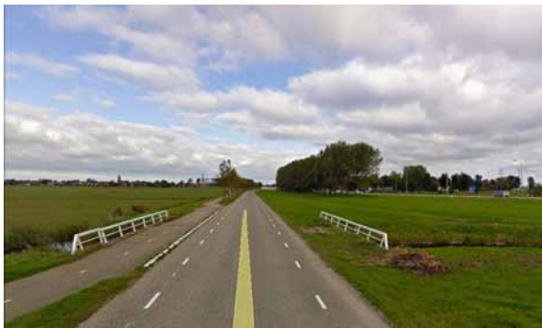
Autobrug in N31 over waterloop
