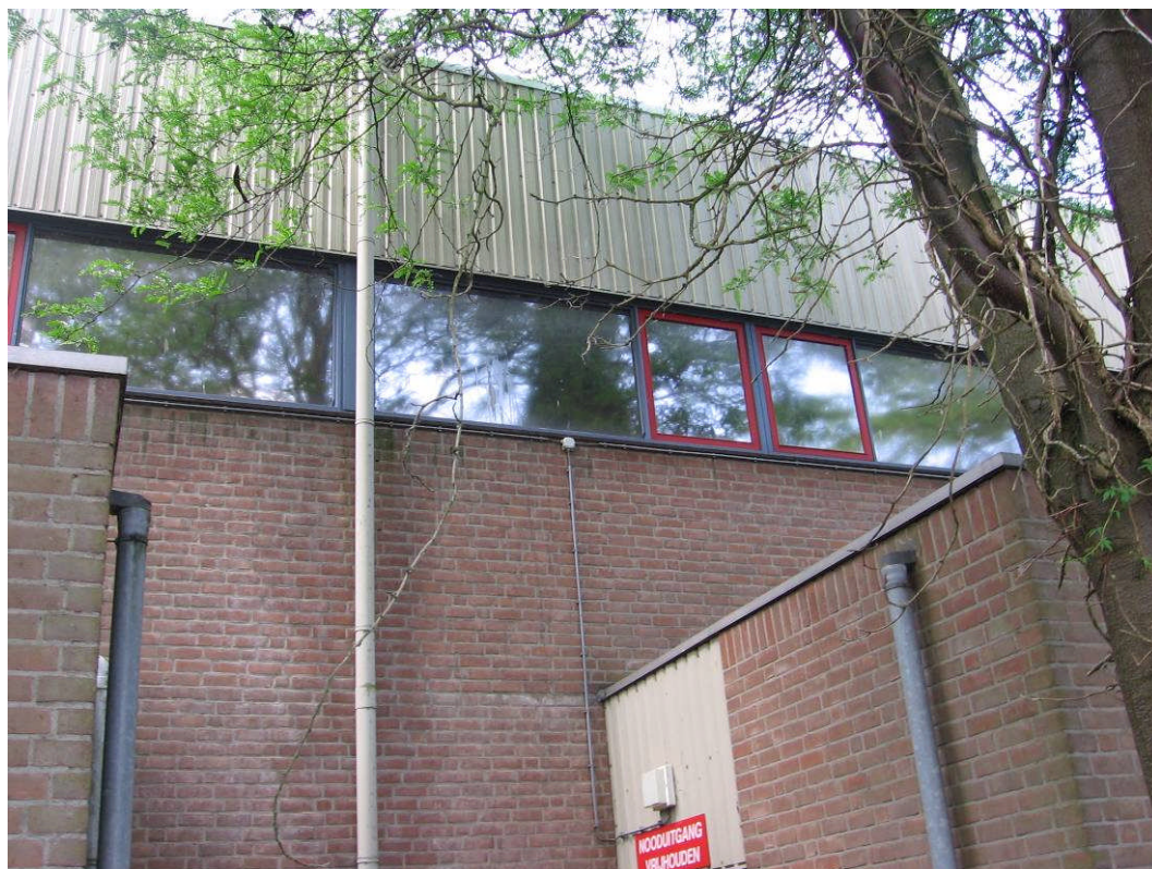
Foto 7: detail langsgevel sporthal
