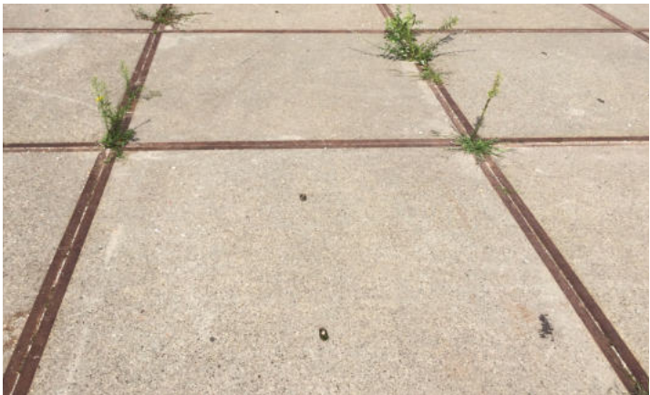
betonplaten (2m*2m) langs de kade
