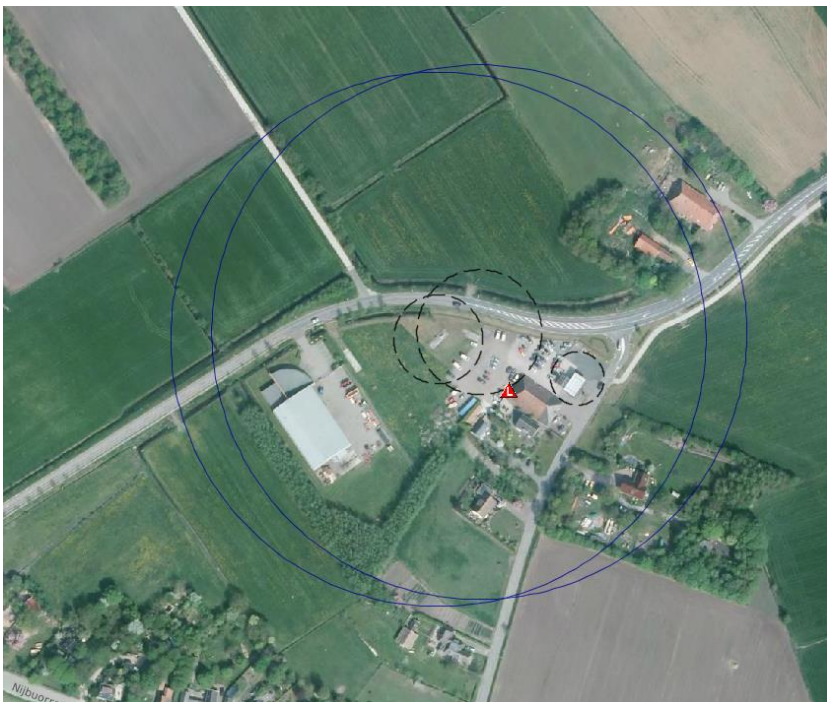
Figuur 13: Nijbuorren 23 in Hemelum, LPG-tankstation Texaco Schilstra
