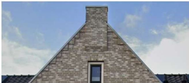
Detailtering dakrand
