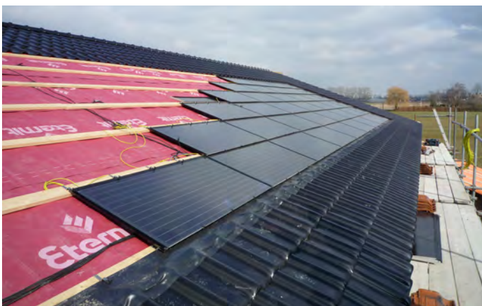
Integratie PV-cellen in dakvlak
