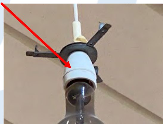
Foto 35 | Pakking fitting hanglampen
