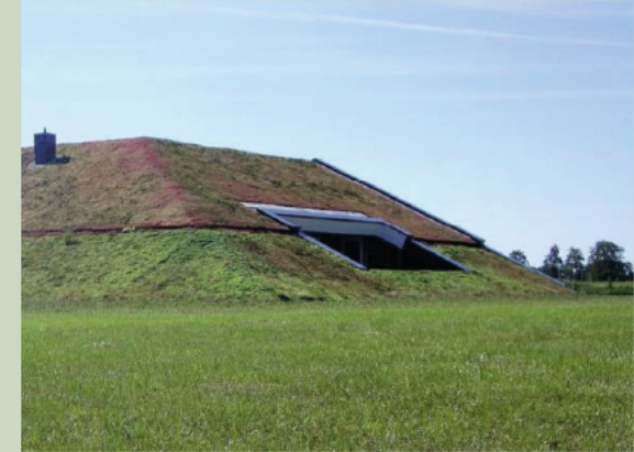
Sedumdak overgaand in grasdak
