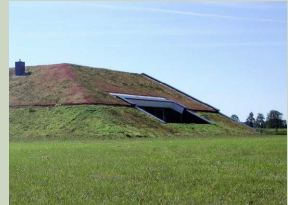
Sedumdak overgaand in grasdak
