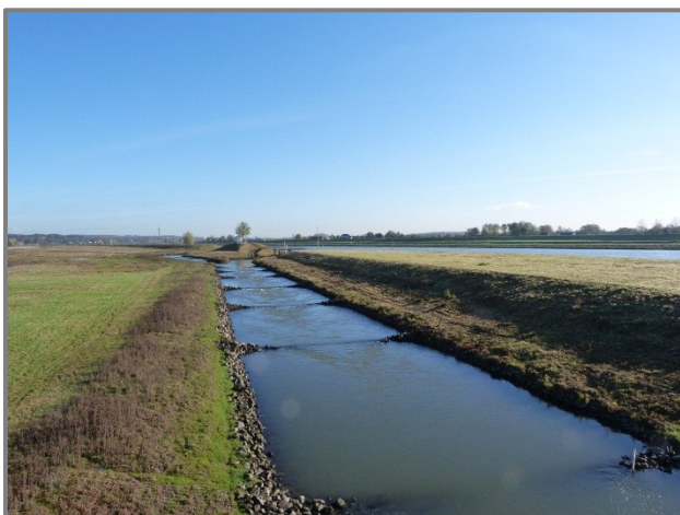
Vistrap stuwcomplex Driel
