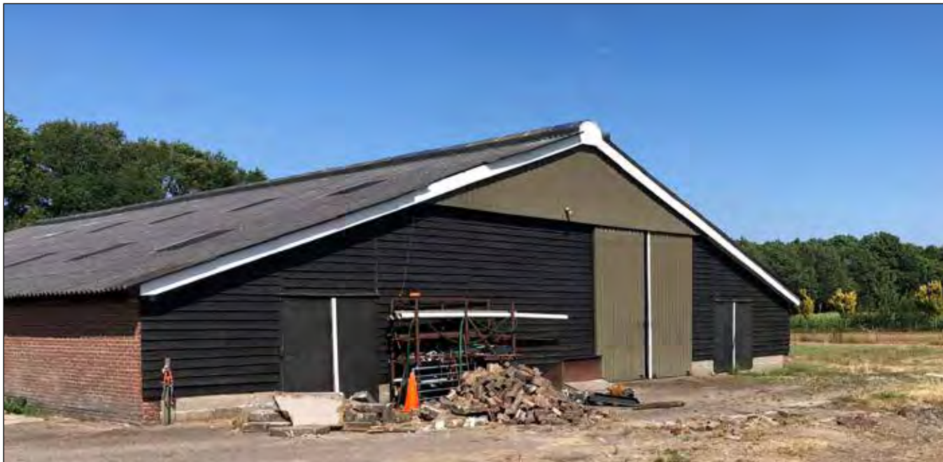
te slopen ligboxenstal
