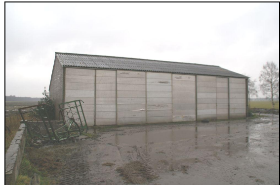
Foto 2. Te slopen machineberging.
