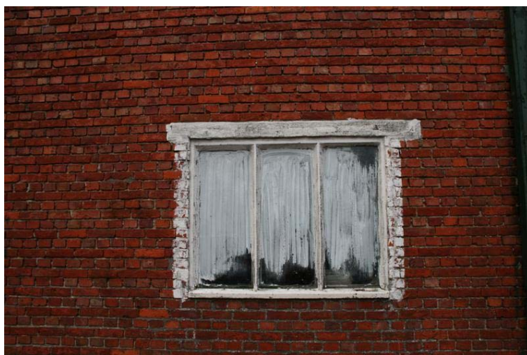
Later aangebracht stalraam
