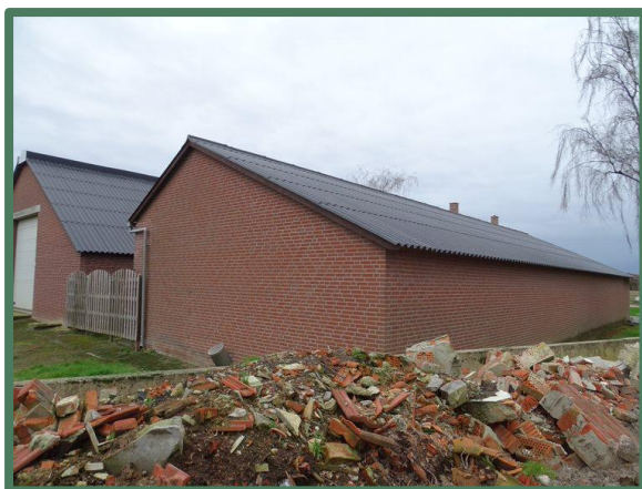
Foto 23: Bouwafval in sleufsilo 22 november 2024
