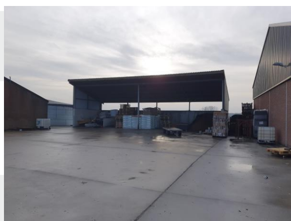
Open loods Markweg 13: open karakter. Golfplaten dakbedekking.
