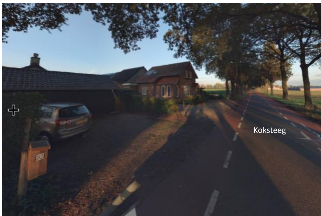
Koksteeg 32 (bron: Streetsmart/Cyclomedia)
