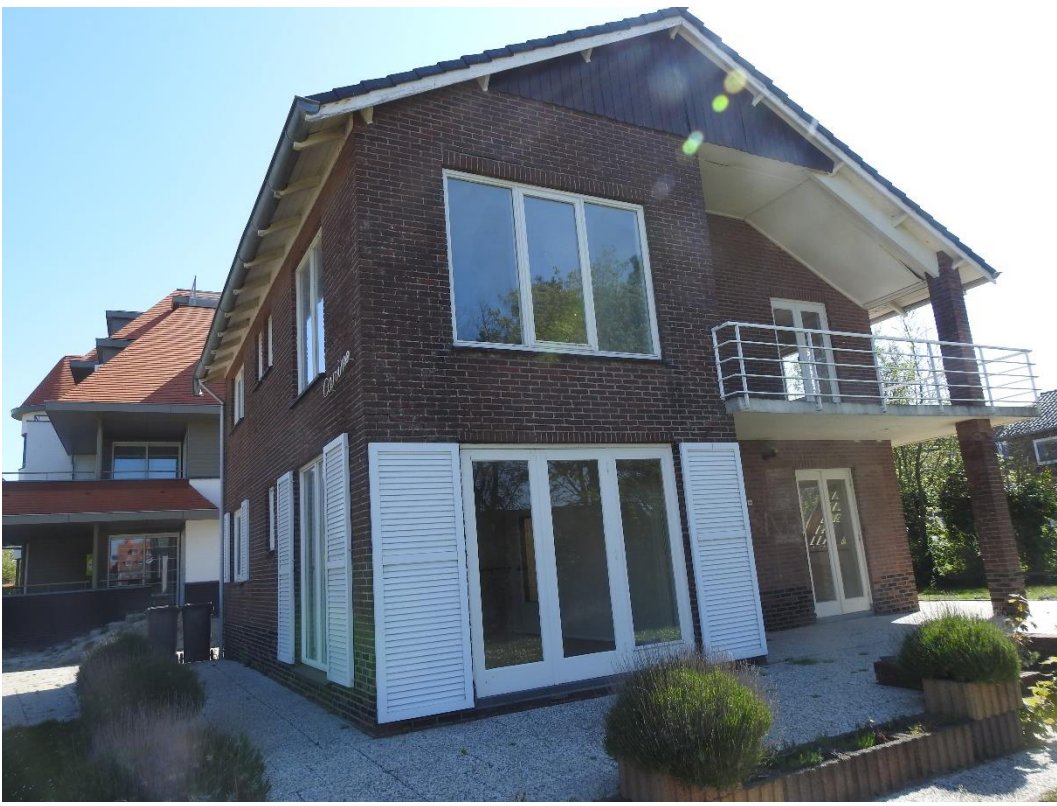
Foto 1. Te slopen woning.
