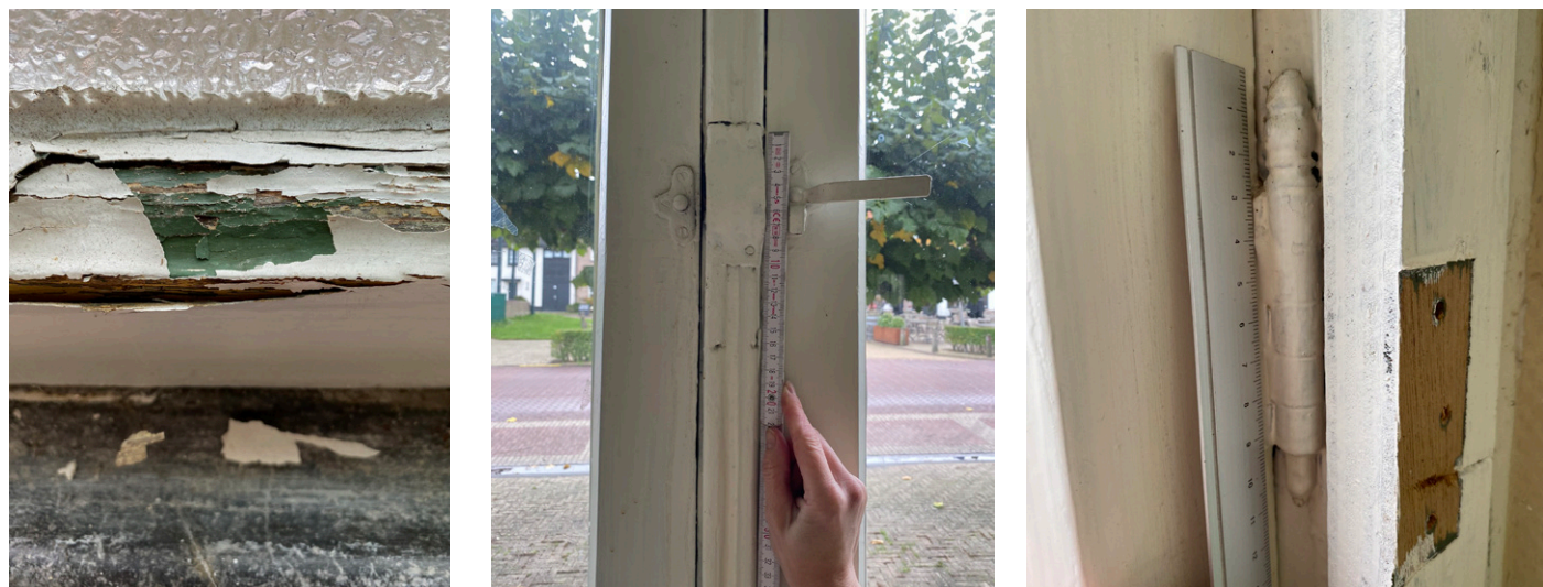
^ detailfoto's origineel houten raam
