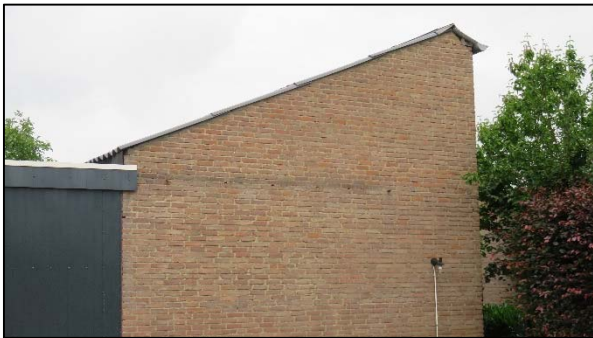
Foto 3. Te slopen loods
