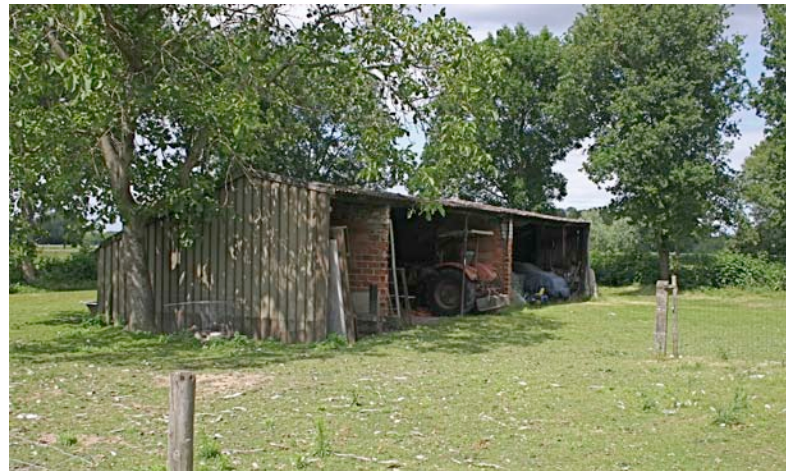
te slopen berging
