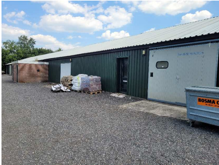
Foto 1 Te slopen loods
