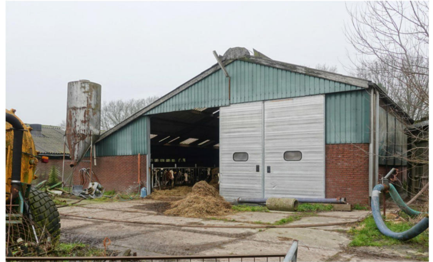
Te slopen stallen
