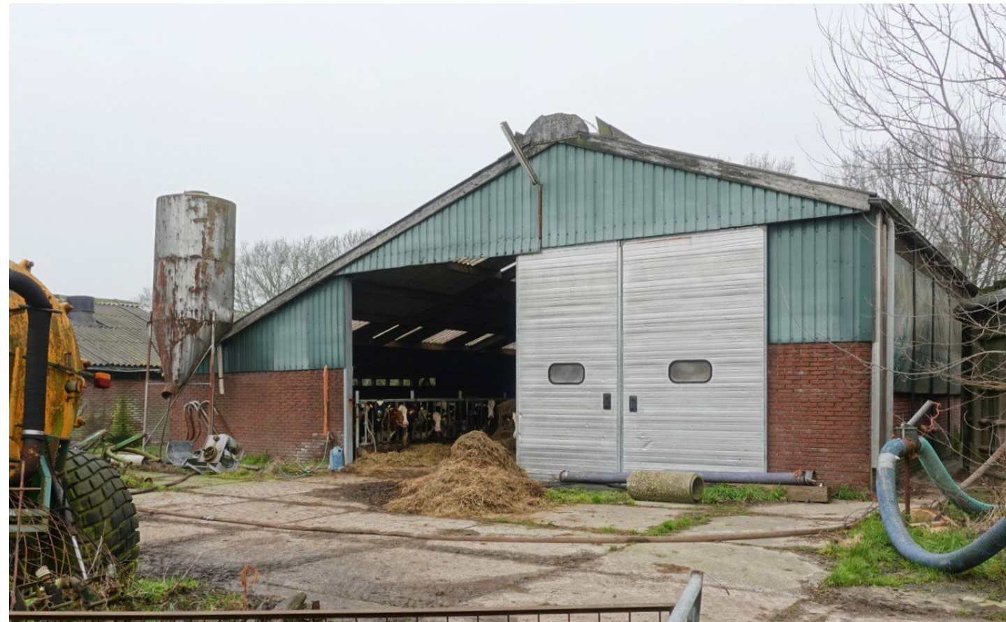
Te slopen stallen
