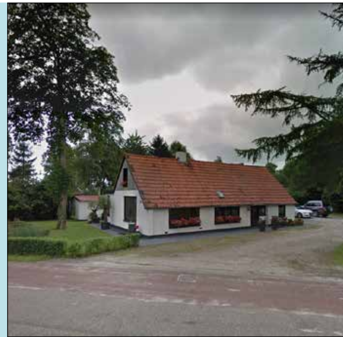
te slopen woning
