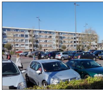
te slopen flat (fase 4)
