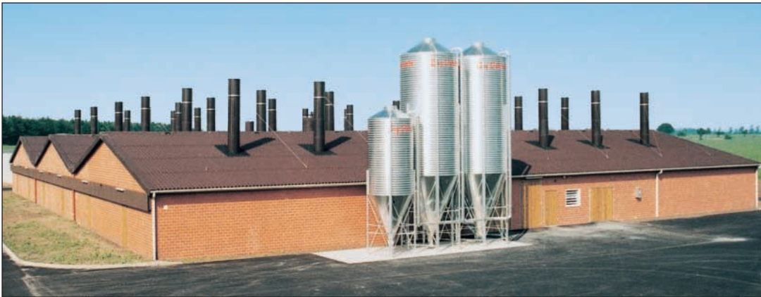
Decentralized exhaust air guiding
