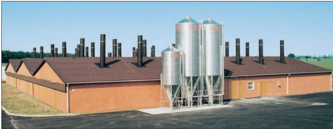
Decentralized exhaust air guiding
