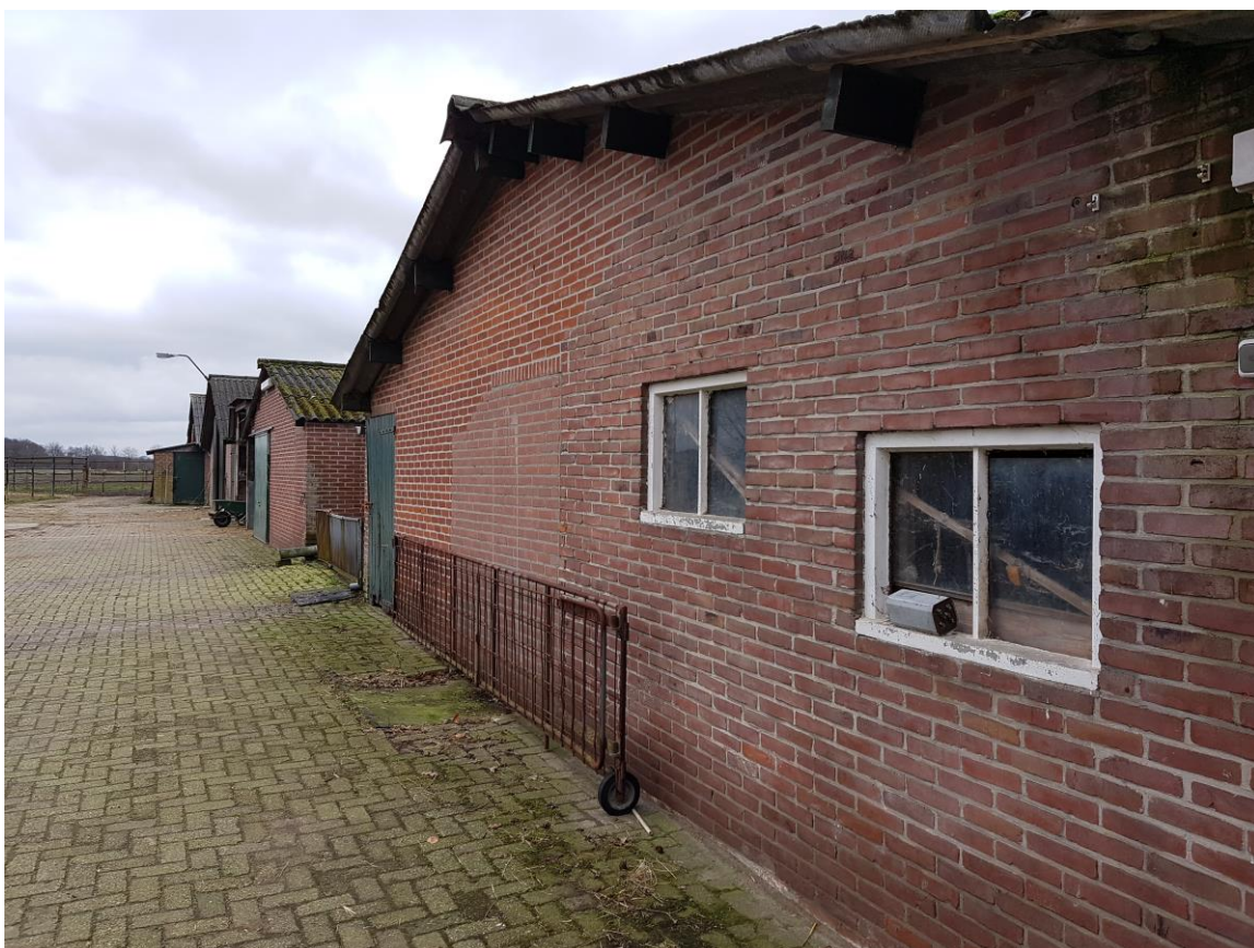
Te slopen stalen
