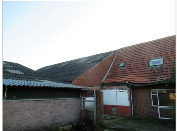
golflaten dak dak no. 5 (foto 2021)
