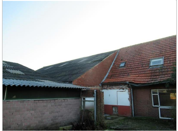
golflaten dak dak no. 5 (foto 2021)
