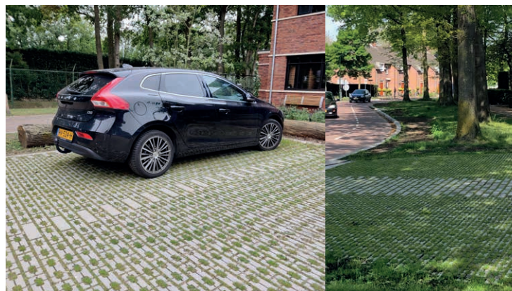
Parkeren in halfverharding
