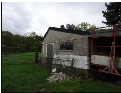
Figuur 3. De te slopen loods.
