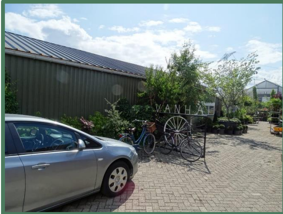
Loods van sandwichpanelen
