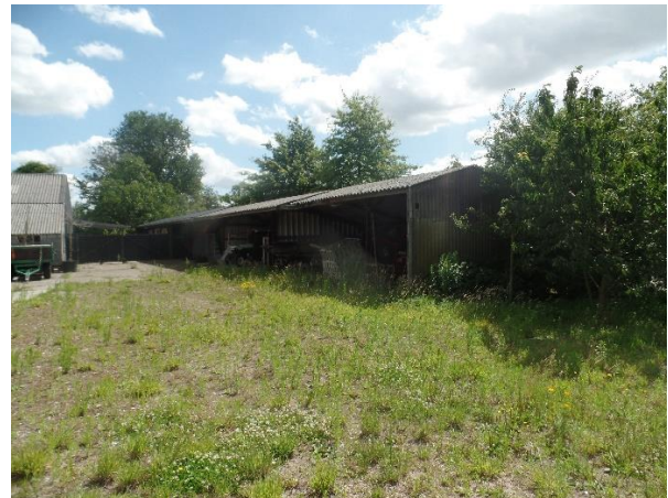
De te slopen lage loods
