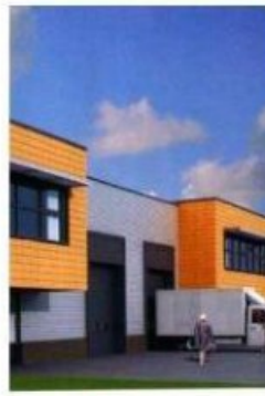
Interne loading docks
