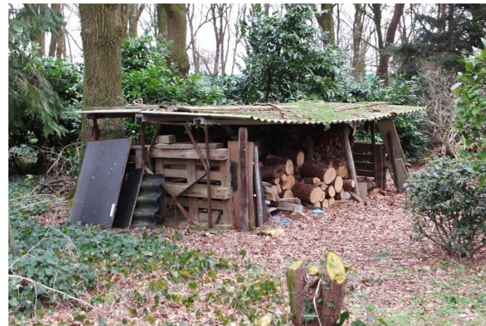
Te slopen houten hokje ± 10m 2
