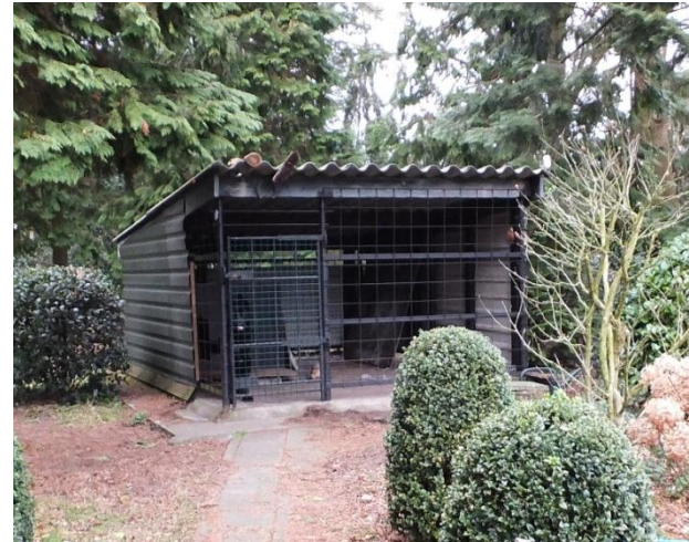
Te slopen hondenhok ± 9,4m 2
